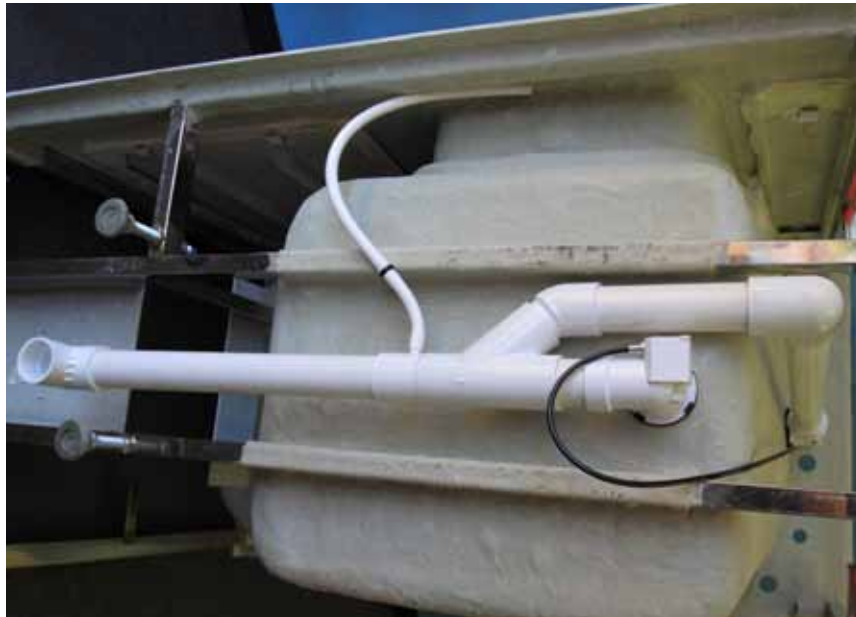
Photo: Reverse Drain Plumbing Installed
